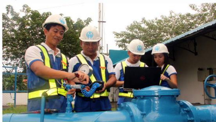
LARC employees install data logger for pressure and flow monitoring at Vega Pump Station, Batong Malake, Los Baños, Laguna.
