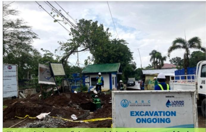
Water service is temporarily interrupted during the improvement of Cambatoc Bridge in Paciano Rizal, Bay on March 8, 2021 due to the relocation and replacement of LARC pipe lines to keep abreast with the wider and better bridge.
