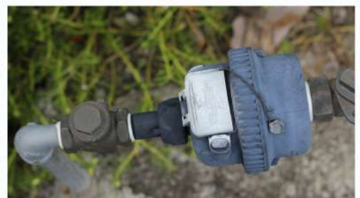
Sample of a newly installed water meter.
