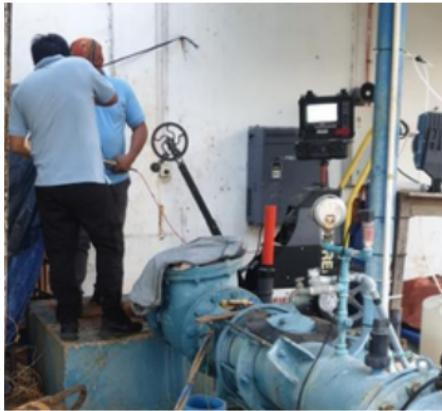
Water well contractors investigate the status and possible cause of sand intrusion at Jubileeville Pump Station on June 13, 2023.
